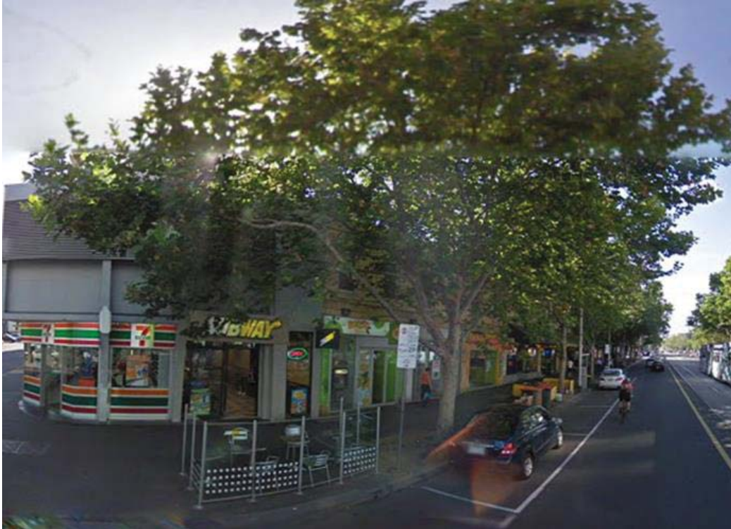
Figure 3 – Site Photo – opposite side of Elizabeth Street – 463 Elizabeth Street Melbourne (Source – Google Maps)
