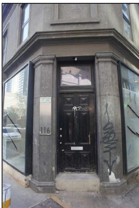
Figure 7 Corner entry and stone pilasters
