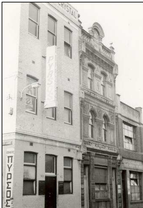
Figure 39 Leitrim Hotel as part of a building group: Karl Halla` 1960 - 1970. Little Lonsdale Street between Russell Street and Exhibition Street (North Melbourne Library)
