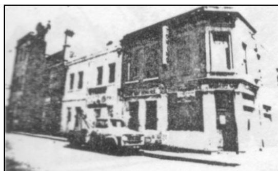
Figure 22 Streetscape 7 showing former ground level of the Exploration Hotel (HBPC study 1976)
