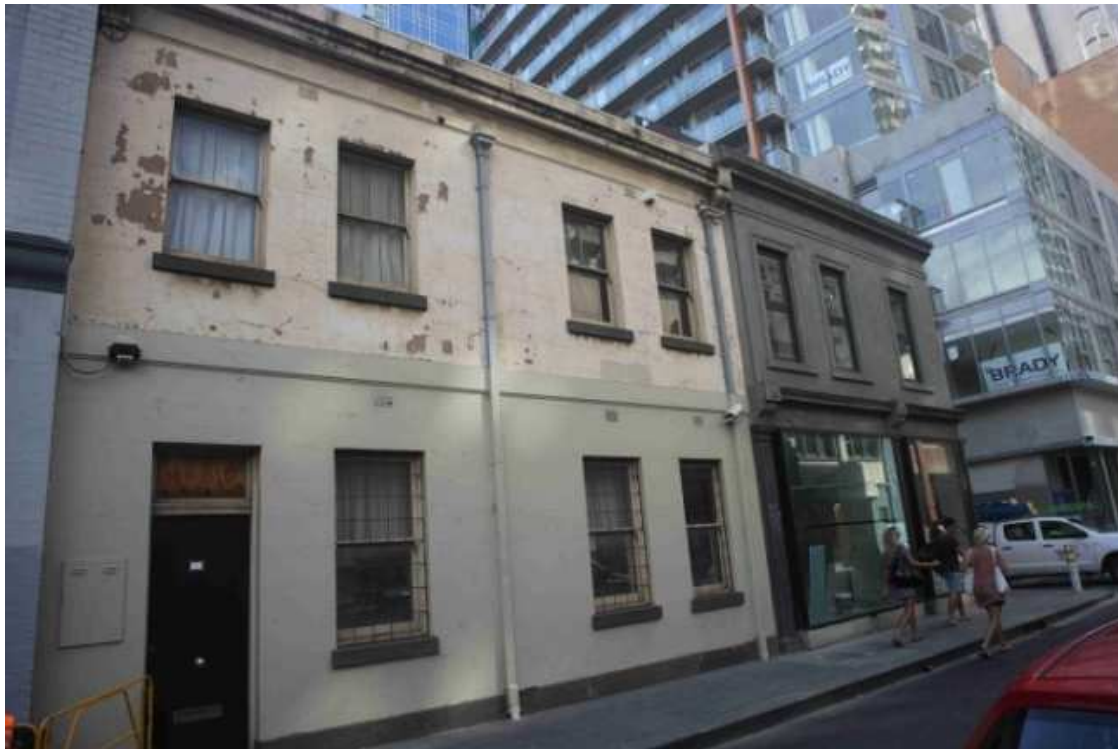
Figure 8 120-122 Little Lonsdale Street, 2010: showing the only major change as conversion of the door of 120 to a matching window when the houses were united.
