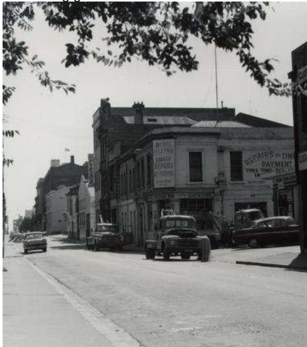
Figure 33 Figure 34 Building group by Karl Halla, 1960 - 1970. Little Lonsdale Street between Russell Street and Exhibition Street ' showing Perlow Motors occupying the former Exploration Hotel (North Melbourne Library)
