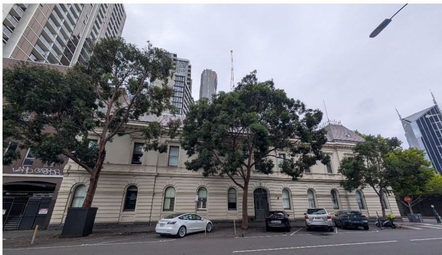
Site Photograph of Indigo Loft Apartments immediately south across MacKenzie Street, captured 03-Apr-26
