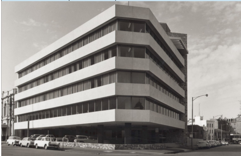
Figure 1: 1963 photograph looking northeast to subject site and newly-completed IOOF Building. (Source: State Library of Victoria, Wolfgang Sievers, 'IOOF Building cr. Russell and Victoria Street, Melb.', Accession No. H2003.100/635)
