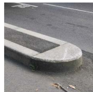
Concrete separator island
