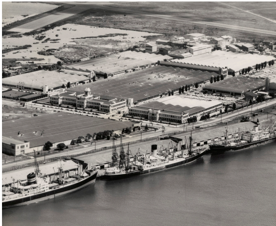
Image 19: Aerial view of Fishermans Bend and Port Melbourne looking south, with ships and General Motors Holden, 1950s, courtesy of the State Library Victoria
