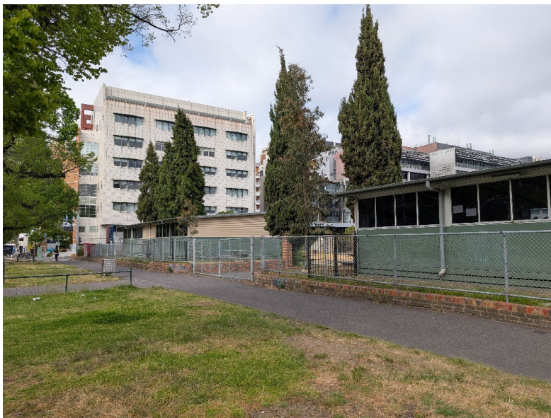
Figure 21 Royal Parade frontage of the oval, looking south-west, entry mid-view Source: Lovell Chen, 2025
