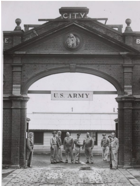
Figure 17 American soldiers at the Royal Parade entry to the school site (temporary army camp), 1941-47 (demolished) Source: State Library of Victoria, H2000.200/1245
