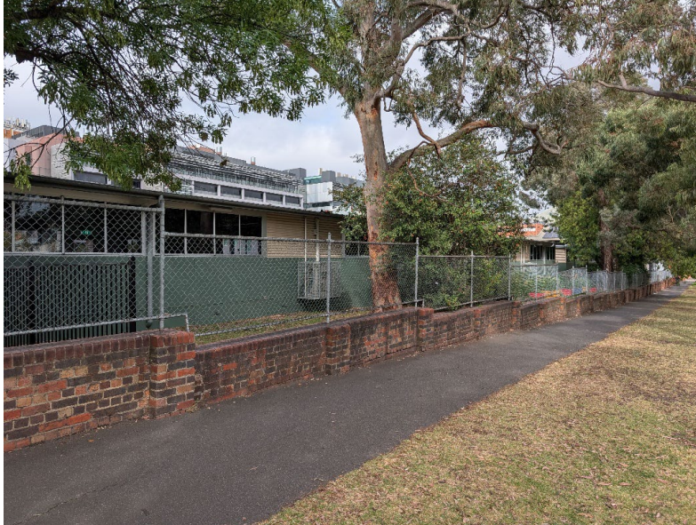
Figure 20 Demountables and rebuilt retaining wall on the Story Street frontage of the oval, view looking west Source: Lovell Chen, 2025
