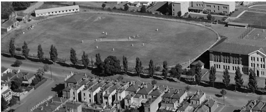
Figure 19 Detail of the 1948 Airspy view, the retaining wall on Story Street is still in place in this view
