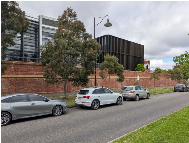
Figure 27 VHR-registered Northern Market wall on Story Street, west of University High School Source: Lovell Chen, 2025
