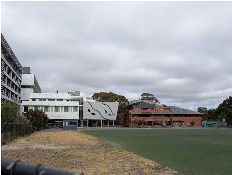
Figure 23 View west across the southern part of the oval Source: Lovell Chen, 2025
