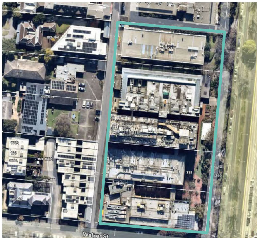
Figure 1 – Monash University Parkville Campus (aerial view)
