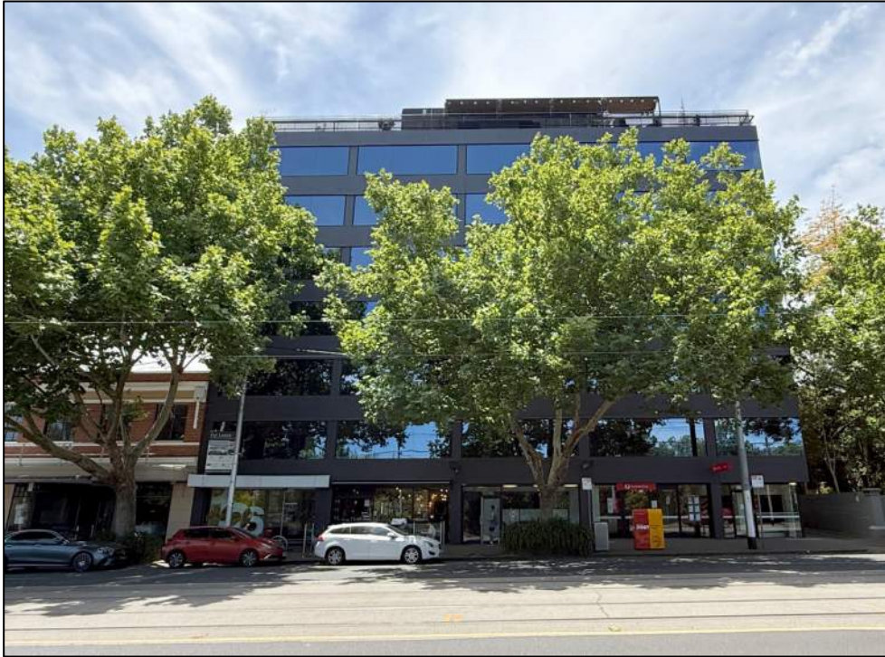
Figure 1 View of the existing building at 122-130 Wellington Parade from the south.
