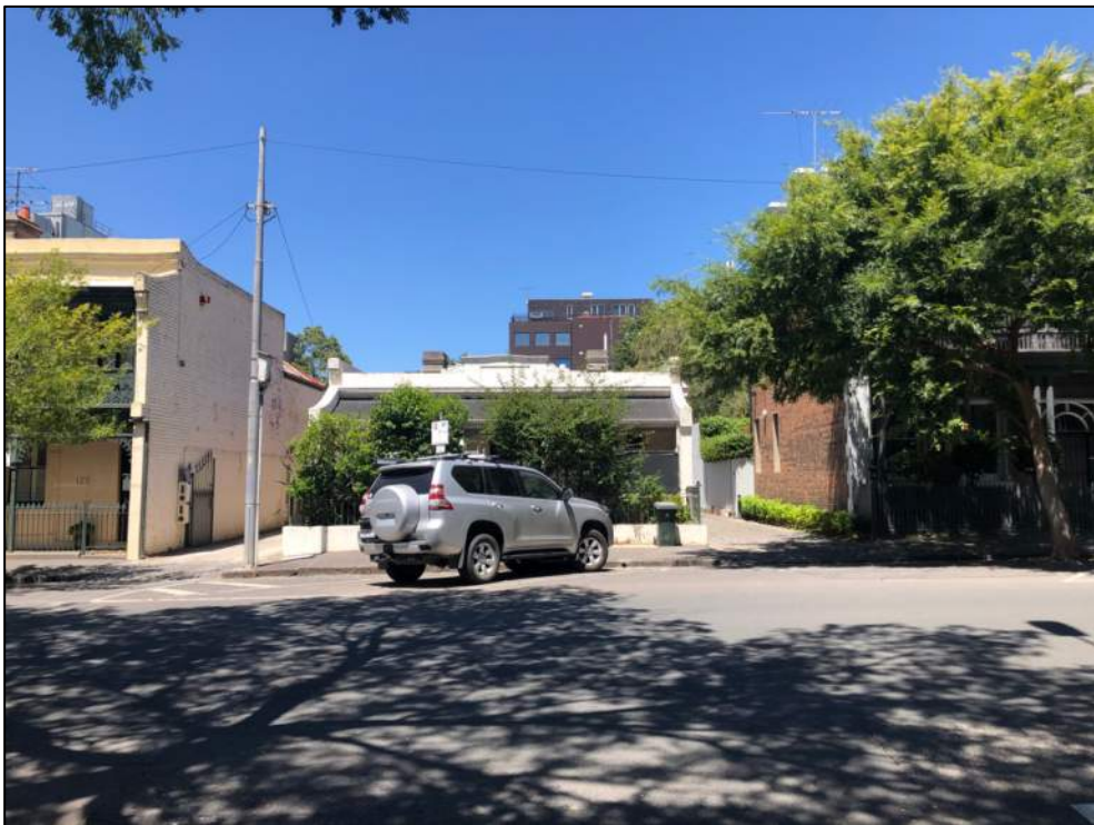
Figure 4 125 George Street (at left), 129 George Street (centre) and 133-5 George Street (at right). The rear of the subject building is visible at some distance beyond.
