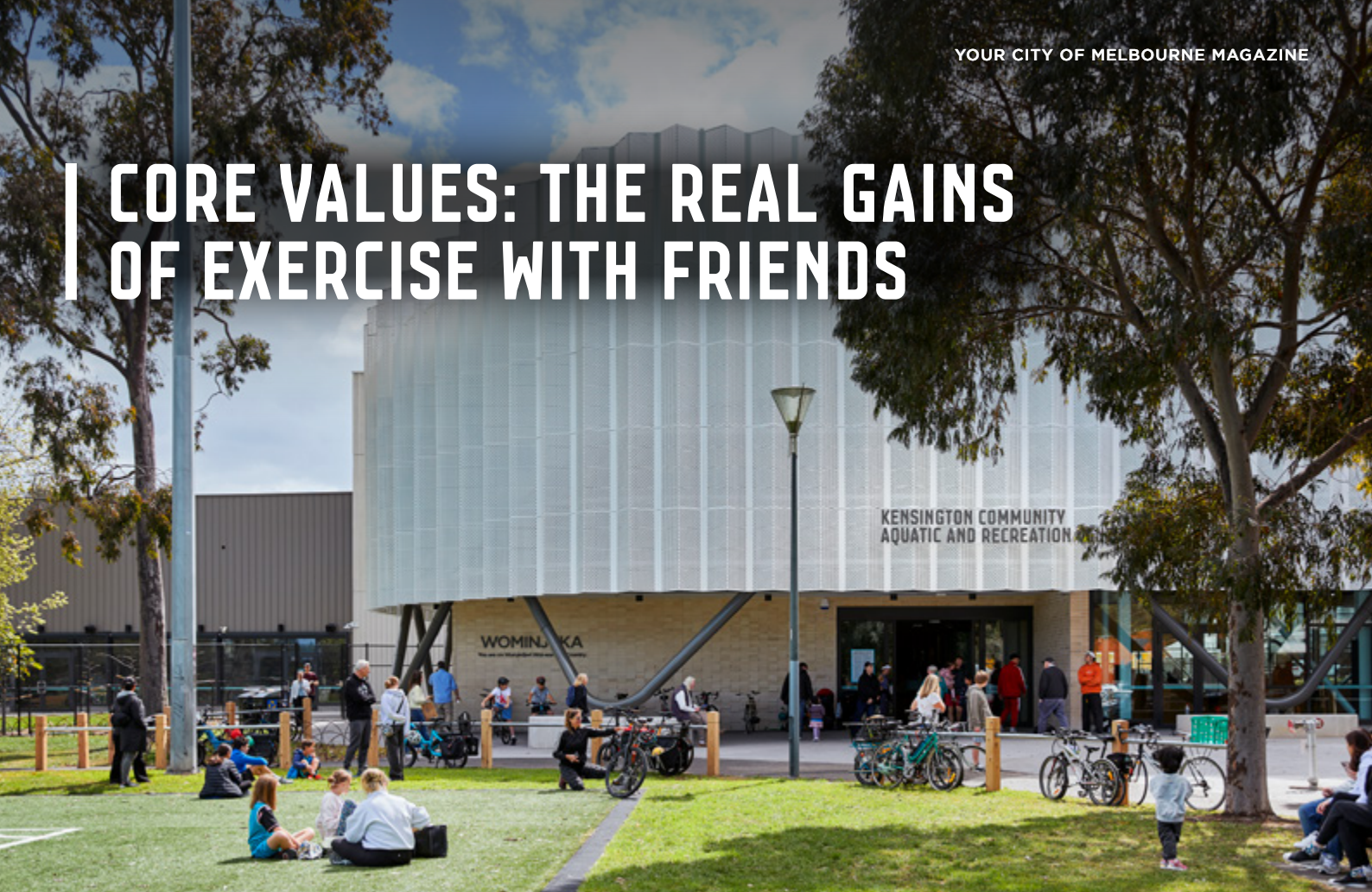
Kensington Community Aquatic and Recreation Centre
