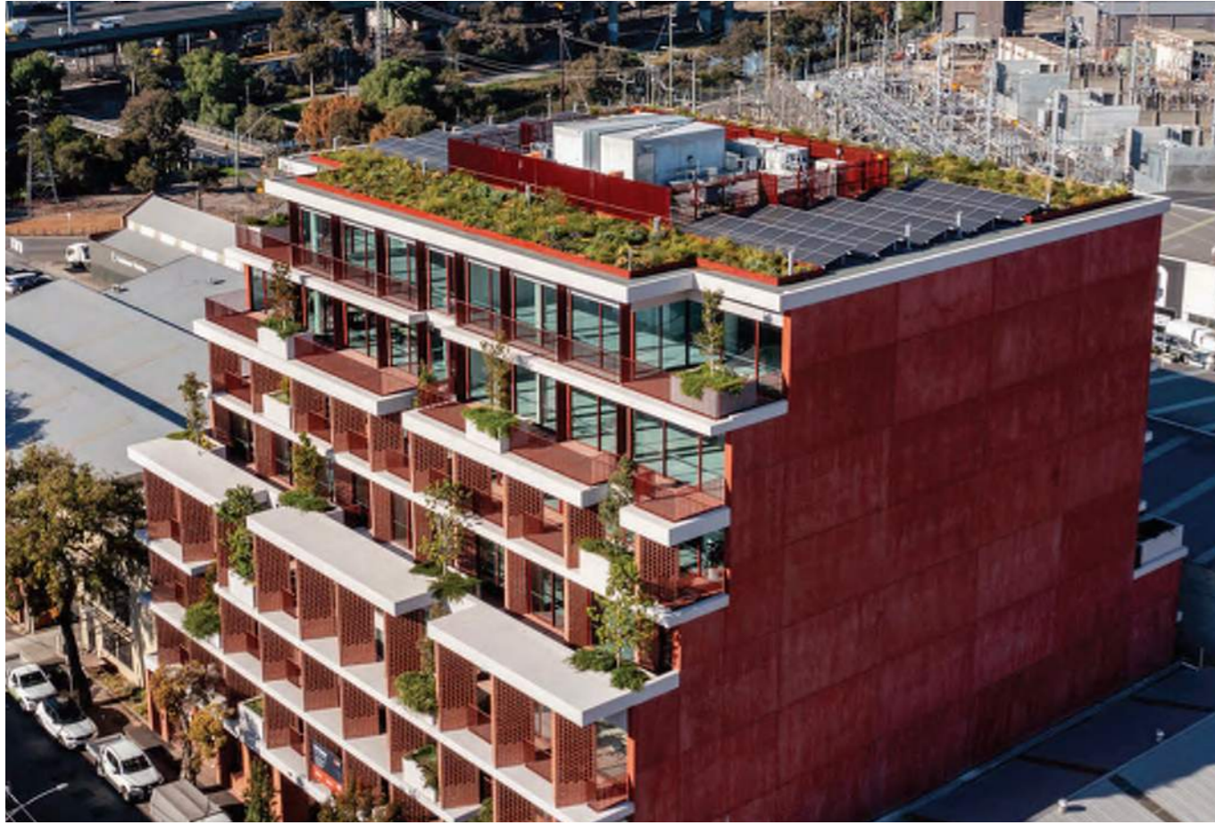
Image 2 Oblique aerial to south-east
