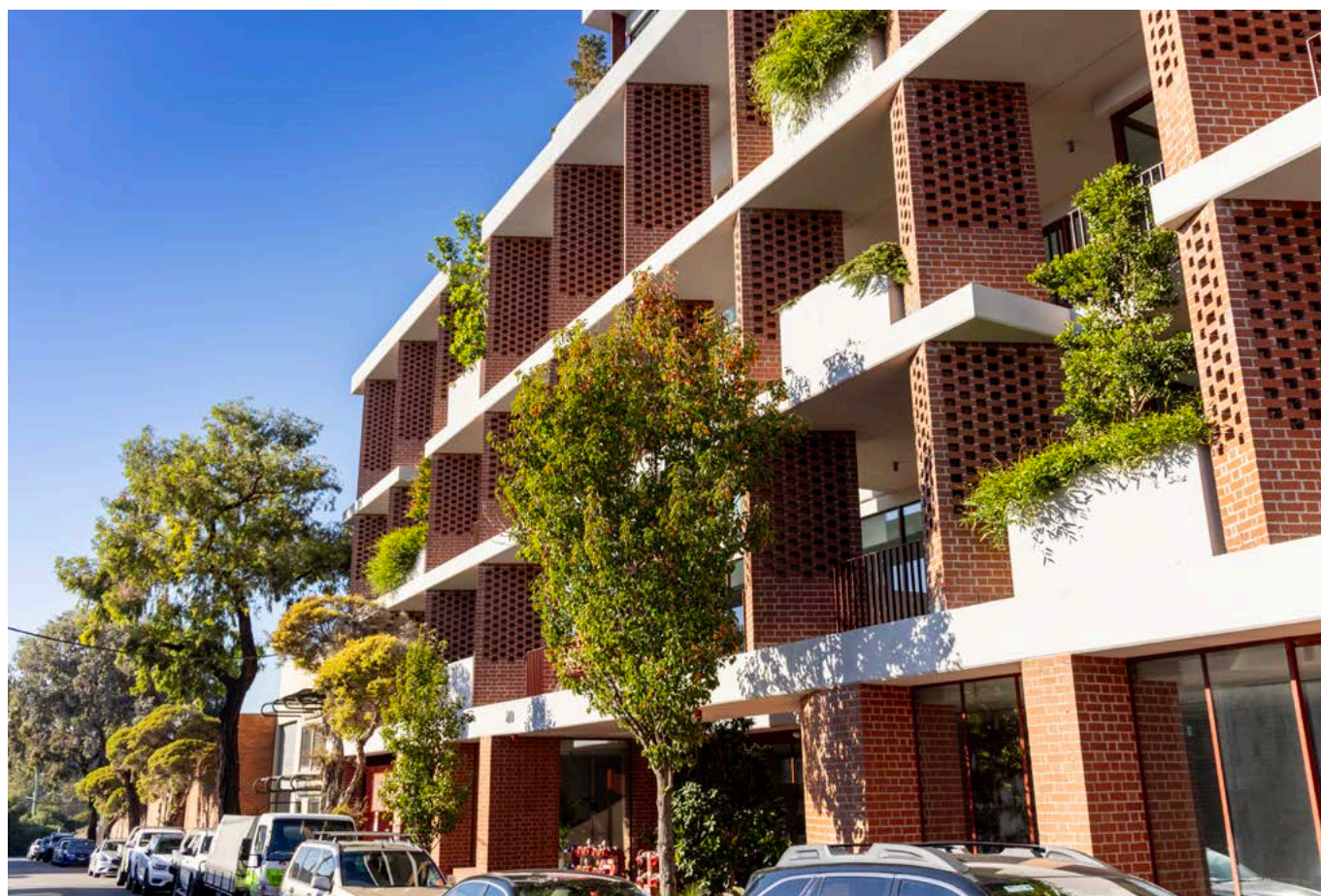
Street view of north elevation showing integration of green infrastructure into the building façade.
