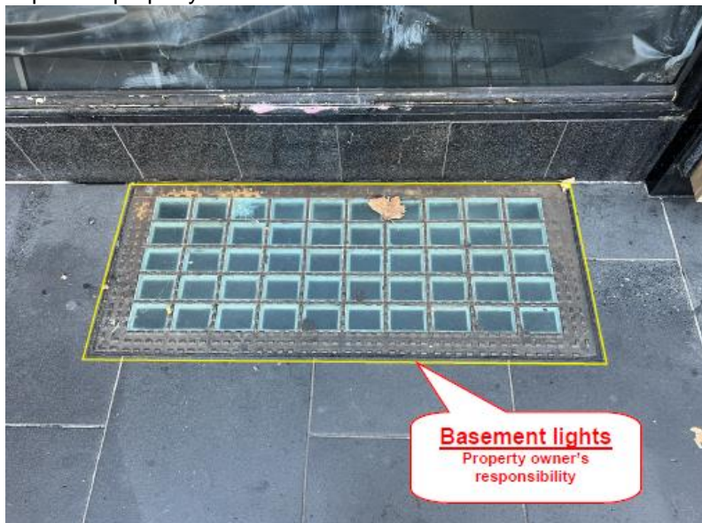
Example of a basement light well
