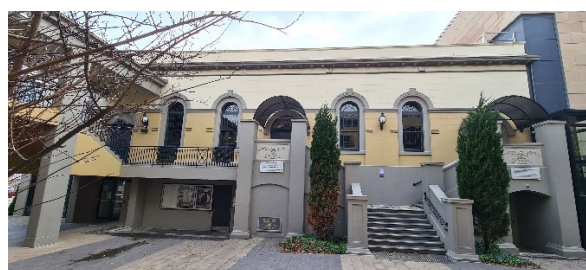
Figure 27. Southern elevation of Adamson Hall. (Source: GML Heritage 2021)
