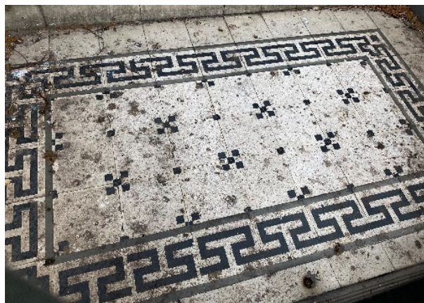
Figure 12. Detail of the tiled threshold with Greek key pattern. (Source: GML Heritage 2021)
