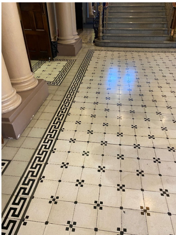
Figure 16. An example of the tiled flooring in the front foyer of the building. (Source: GML Heritage 2021)
