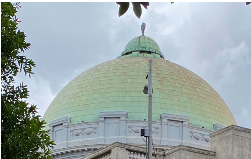
Figure 7. The building's dome, surmounted with cupola and finial bearing the Star of David. The detailing on the drum of the dome can also be seen. (Source: GML Heritage 2021)
