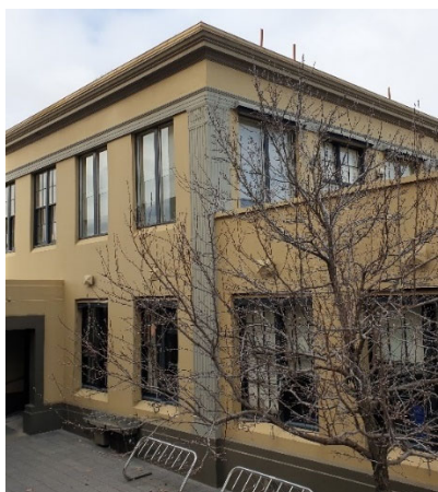
Figure 44. Northern elevation of the Senior School faculty building, showing some of the original multipaned windows intact. (Source: GML Heritage 2021)
