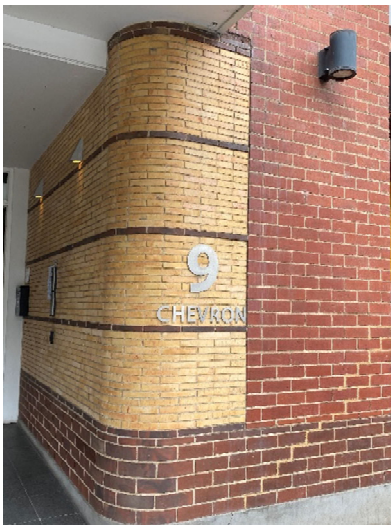
Figure 10. The formal entry of the 1934 portion fronting Commercial Road, finished with brown and red bricks with decorative cream and brown roman bricks. (Source: GML Heritage 2021)
