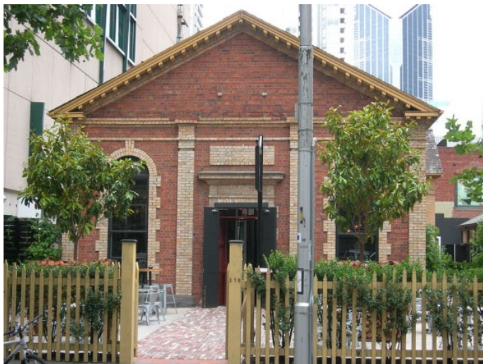
Figure 25. Former Mickveh Yisrael Synagogue, 275–285 Exhibition Street, Melbourne, built in 1859. (Source: Victorian Heritage Database)
