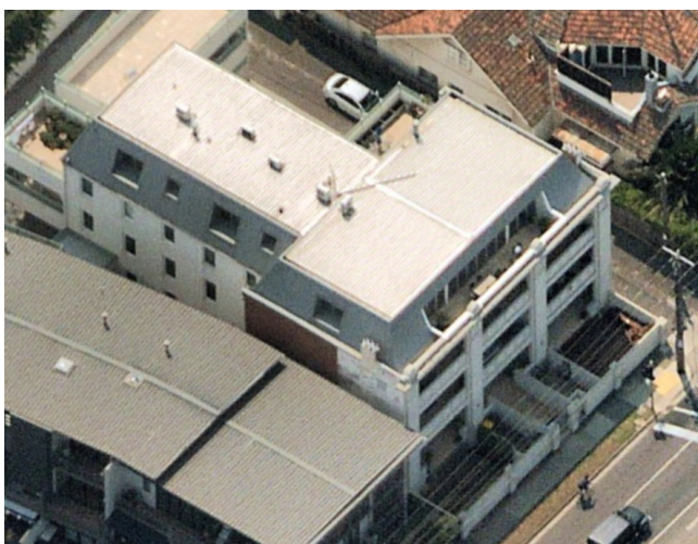
Figure 17. 65 Ormond Esplanade, Elwood, built in 1927. (Source: Nearmap 2021)
