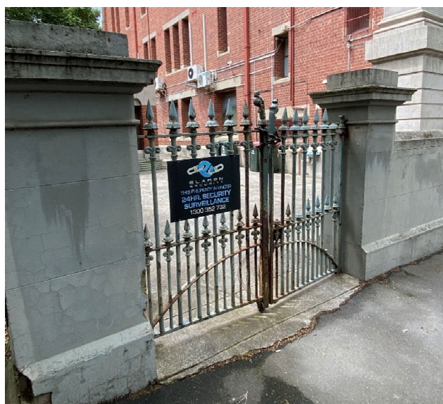
Figure 15. The Victorian gates removed from the original Bourke Street synagogue and installed as part of the perimeter wall on the new site along Arnold Street. (Source: GML Heritage 2021)
