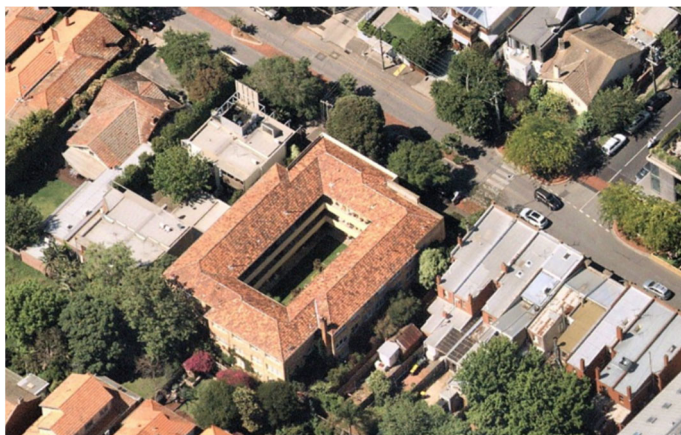
Figure 29. Aerial imagery showing the Merton Court, 169 Ormond Road, Elwood, built in 1951. (Source: Nearnap 2019)
