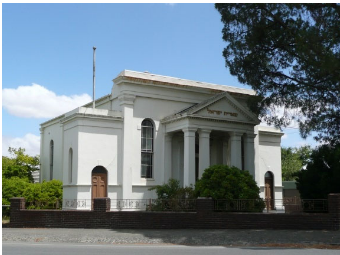
Figure 27. Synagogue, 2–4 Barkly Street, Ballarat East, 1861. (Source: Victorian Heritage Database)
