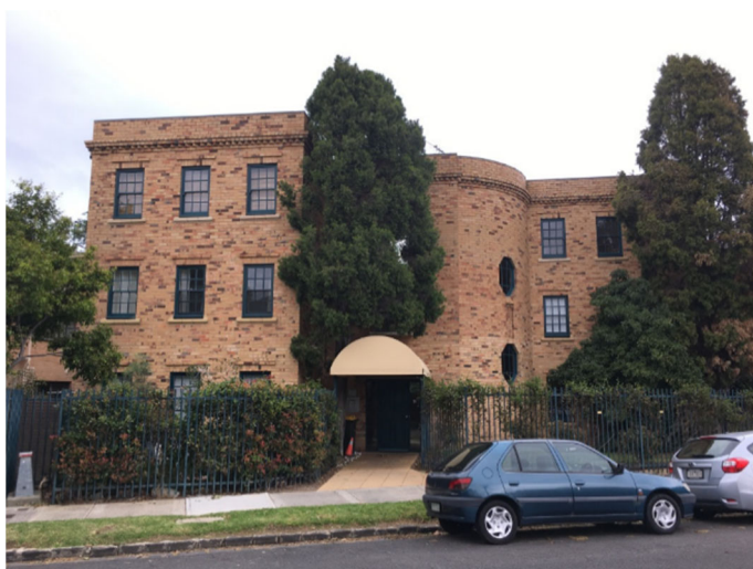
Figure 28. Deansgate, 9 Southey Street, Elwood, built in 1949. (Source: Hermes)
