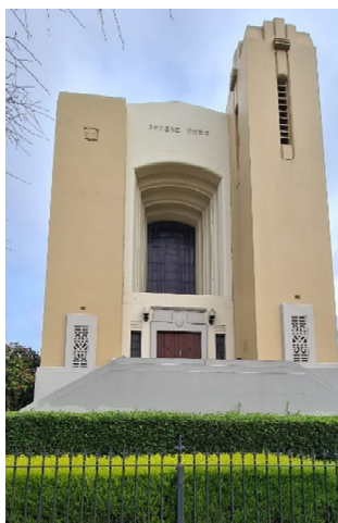
Figure 37. Principal façade of the Chapel, fronting Punt Road to the east. (Source: GML Heritage 2021)
