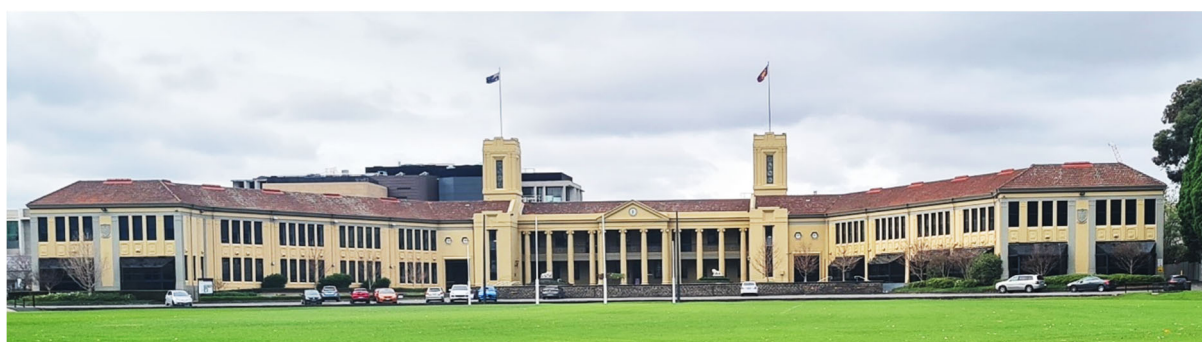
Figure 25. Main building incorporating the Menzies Wing (left) and Holt Wing (right) (Source: GML Heritage 2021)
