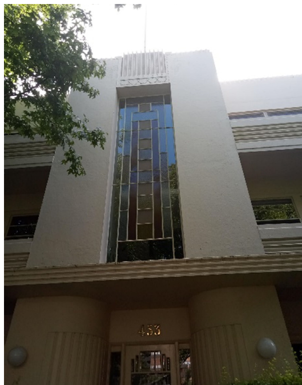
Figure 10. Entrance tower with coloured glass windows. (Source: GML Heritage 2021)
