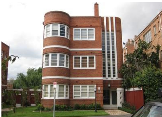
Figure 25. 6 Garden Avenue, East Melbourne, built in 1930. (Source: CoMMaps)
