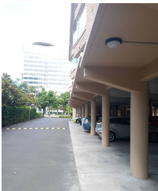
Figure 11. Cantilever from pillar to first floor base on the southern side. (Source: GML Heritage 2021)
