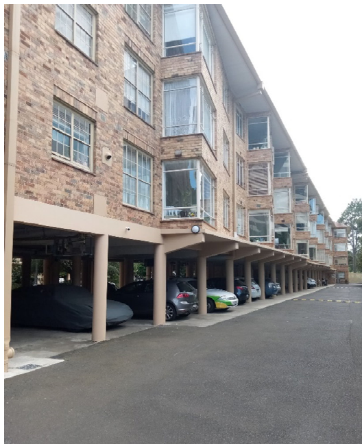
Figure 10. Windows along the serrated southern side. (Source: GML Heritage 2021)
