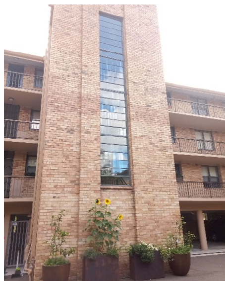
Figure 15. Stairwell at the eastern end of the courtyard. (Source: GML Heritage 2021)
