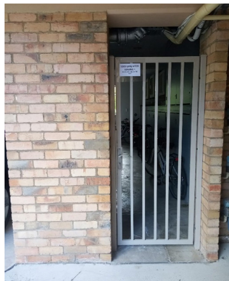
Figure 17. Doorway to bike room. (Source: GML Heritage 2021)
