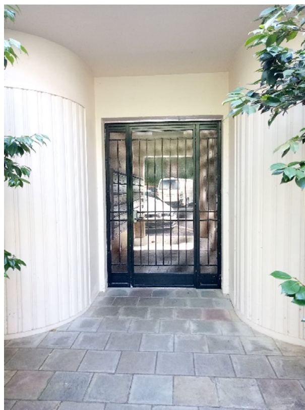
Figure 17. Recessed bay entrance to the carpark with curved walls featuring vertical ribbing. (Source: GML Heritage 2021)
