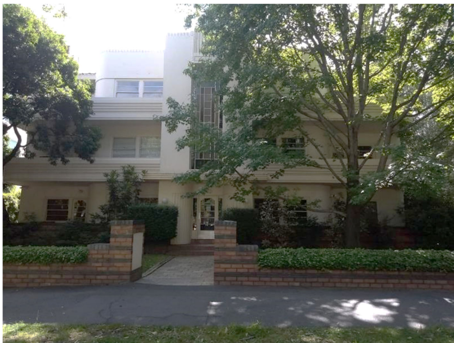
Figure 8. Western façade, facing St Kilda Road, showing front fence with contrasting face brickwork with horizontal stripe patterning. (Source: GML Heritage 2021)
