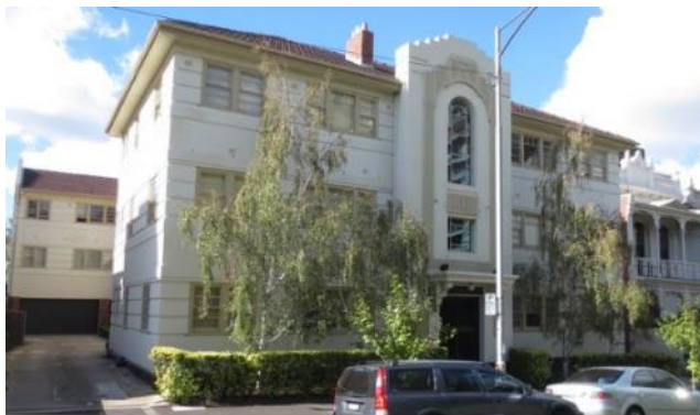
Figure 23. 16–24 Powlett Street, East Melbourne, built in 1935. (Source: CoMMaps)
