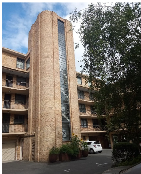
Figure 14. Stairwell at the western end extending above the main building and housing a lift. (Source: GML Heritage 2021)
