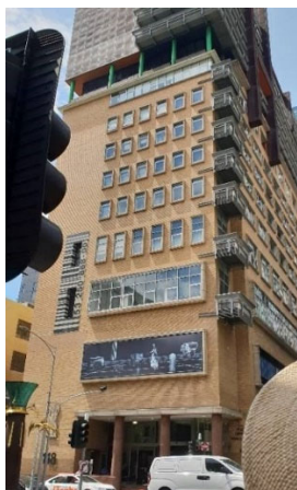
Figure 6. 114–120 Russell Street, built in 1948–154. (Source: Context 2020)
