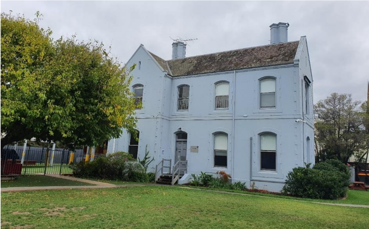
Figure 11. View of the former manse, built in 1873 and added to c1890 (Figure 7: Number 2). (Source: GML Heritage 2021)
