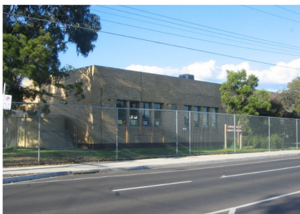
Figure 28. Coburg North Primary School No. 4523, built 1937. (Source: Hermes)
