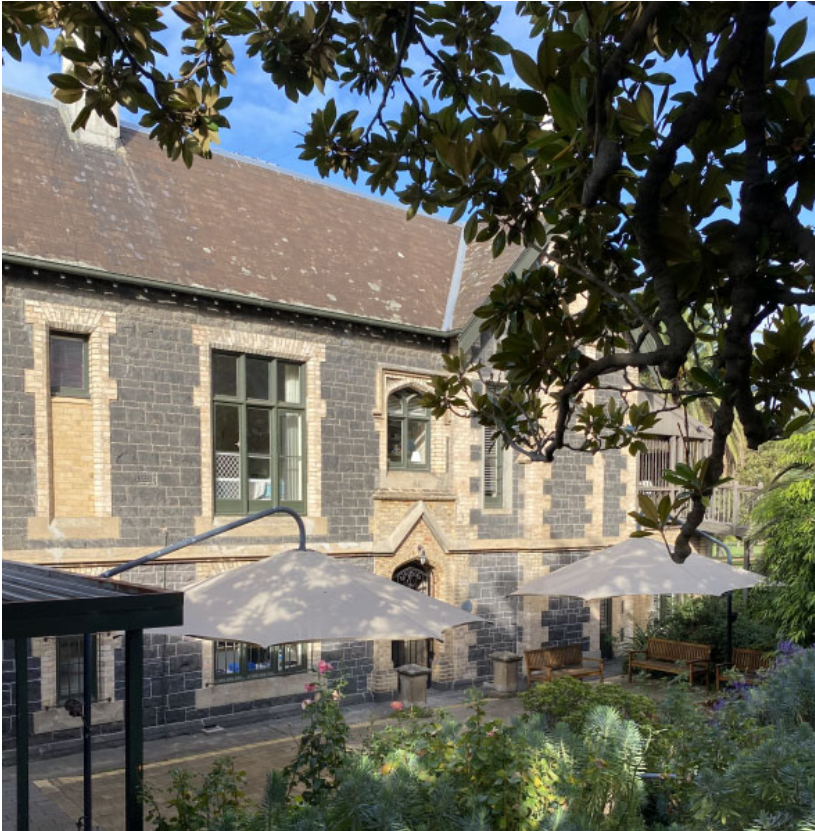
Figure 9. A view of the northern elevation of the Vicarage. The height of the first floor against the ground floor is evident. Note the bricked up window to the left. (Source: GML Heritage 2021)
