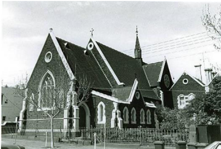
Figure 15. 53–63 Queensberry Street, Carlton, built c1854–65 and altered in 1871 and 1887 to a design by Leonard Terry. (Source: National Trust 1989, via Victorian Heritage Database)
