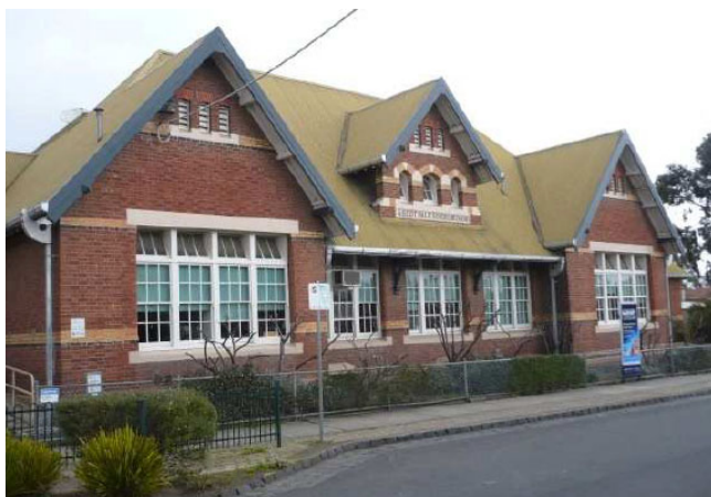
Figure 25. 15–27 Bank Street, Ascot Vale, built in 1901–02. (Source: Hermes)
