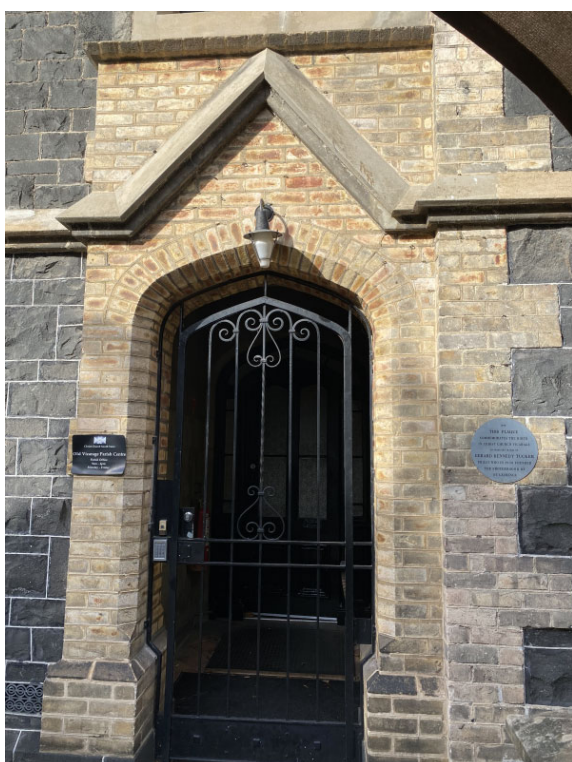
Figure 7.- The recessed porch entry of the vicarage on the ground floor of the northern elevation. (Source: GML Heritage 2021)
