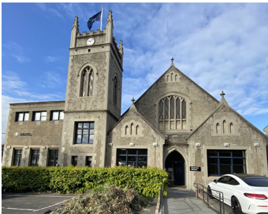
Figure 11. The northern elevation of the Christ Church Hall building. The large gable of the hall is evident with Gothic-style window, with two gabled projecting wings visible at ground floor. The central porch with arched entry is also visible. Note the tower and double-storey wing built in two stages to the east (at the left of the image). (Source: GML Heritage 2020)
