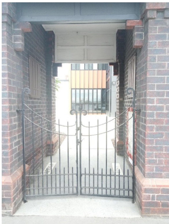
Figure 20. Interior of the Memorial gateway structure. (Source: GML Heritage 2021)
