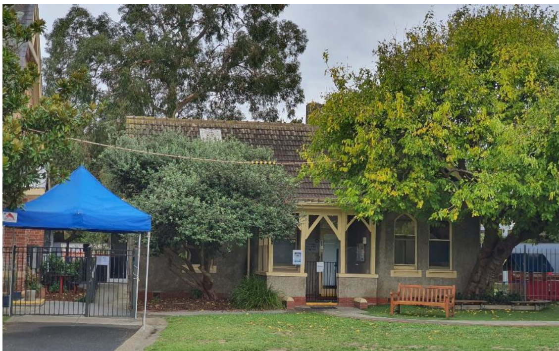
Figure 13. Former caretaker's cottage (Figure 7: Number 6) built in 1925. Note the decorative timberwork to the front porch and the pointed arched windows on the projecting wing on the right-hand side. (Source: GML Heritage 2021)
