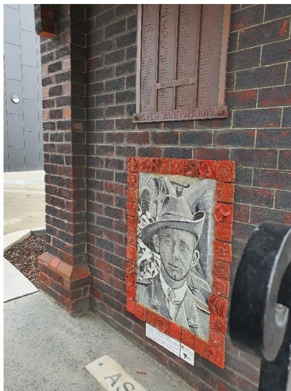
Figure 21. Detail of the memorial gateway commemorative elements. (Source: GML Heritage 2021)
