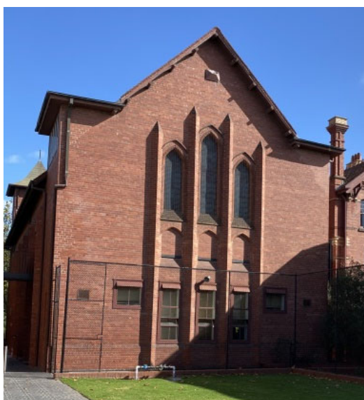
Figure 13. Rear façade of the chapel, facing east. The addition of dormer windows has changed the profile of this roofline, evident in the two horizontal projecting rooflines shown in this picture. (Source: GML Heritage 2021)
