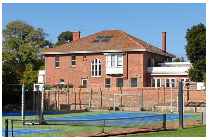
Figure 10. Side elevation of Merton Hall, facing east. (Source: GML Heritage 2021)
