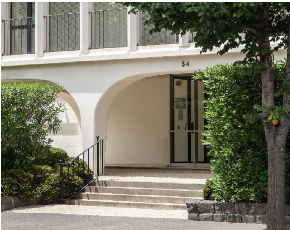
Figure 2. Concrete steps to the entry portico. Note the intact arched pilotis, modular frames and metal balustrading. (Source: GML Heritage 2021)
