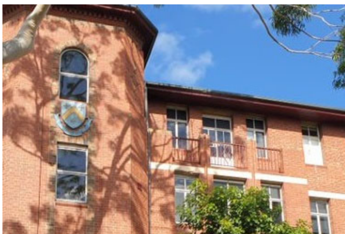
Figure 16. Detail showing dark brown brick detailing and mild steel balcony balustrade. (Source: GML Heritage 2021)
