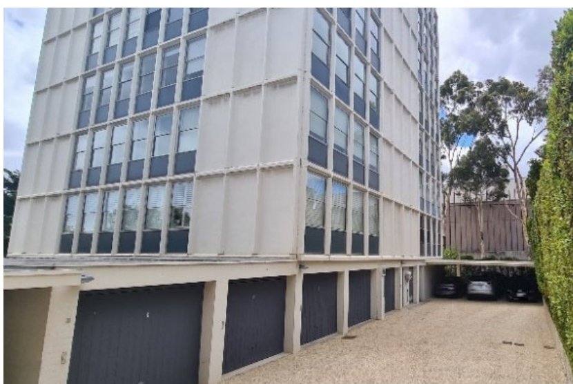
Figure 6. Side and rear elevations comprising 12 bays and incorporating vertical strips of curtain walls. Carports at the rear of the property to the east, enclosed within the brick fence. (Source: GML Heritage 2021)
