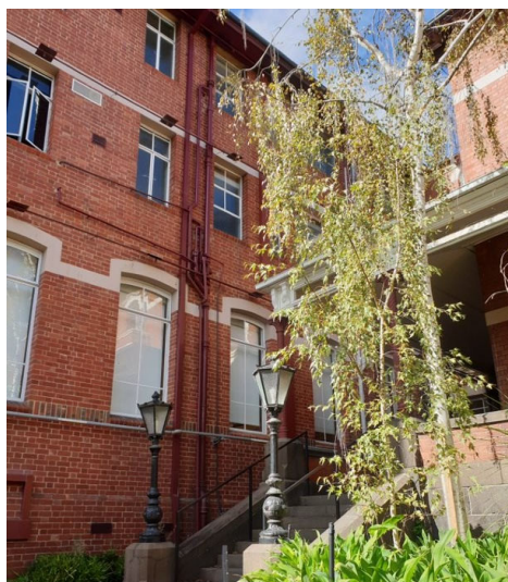
Figure 18. Phelia Grimwade House extension, side elevation facing west. (Source: GML Heritage 2021)
