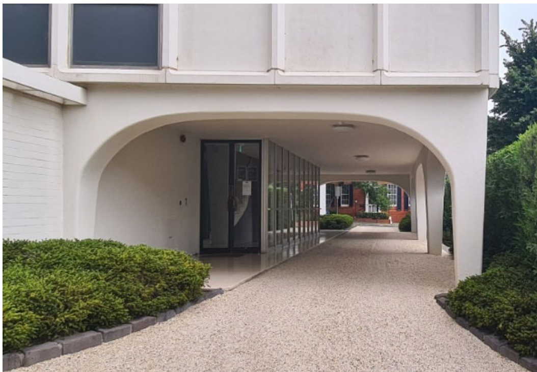
Figure 3. Entry portico. (Source: GML Heritage 2021)
