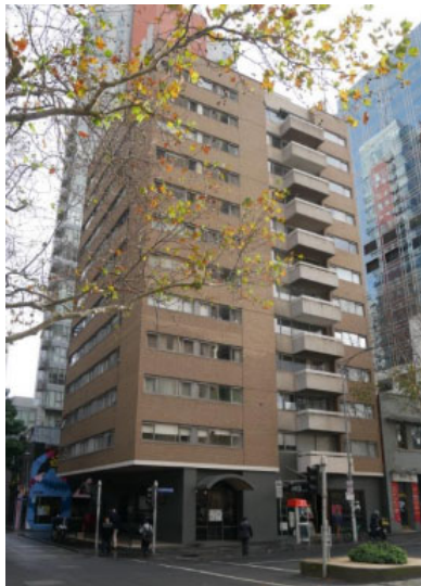
Figure 10. 287–293 Exhibition Street, Melbourne, built in 1969–71. (Source: GJM Heritage 2020)
