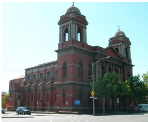
Figure 13. Former Church of the Sacred Heart, 169–199 Rathdowne Street, Carlton, built in 1897–99. (Source: Victorian Heritage Database)
