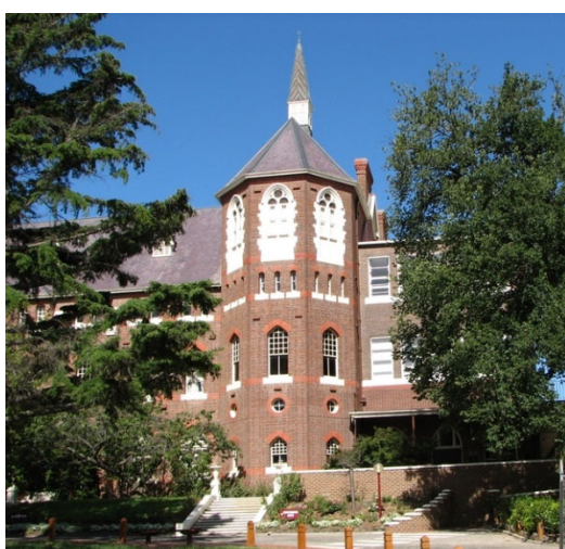
Figure 26. Genazzano FCJ College, 285–315 Cotham Road, Kew. (Source: Heritage Victoria 2008 via Hermes)
