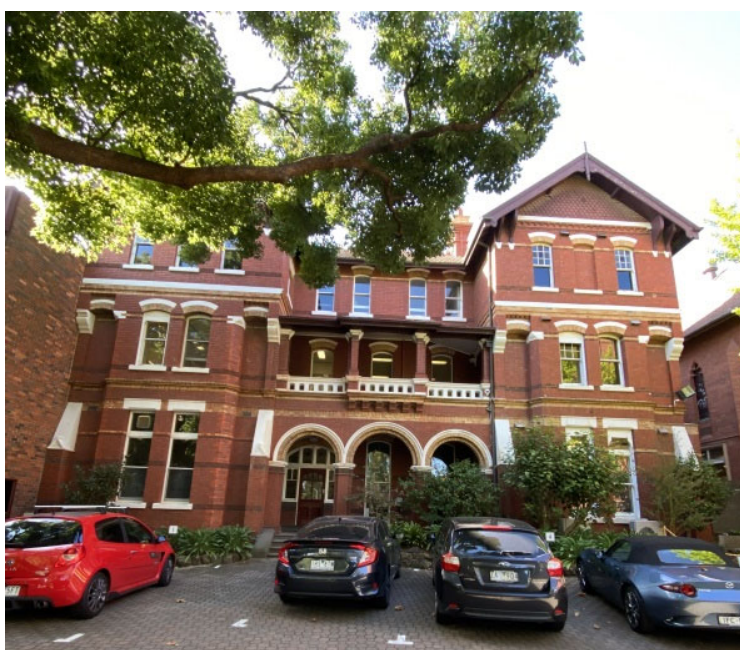
Figure 6. The principal (west) façade of the Merton Hall. (Source: GML Heritage 2021)
