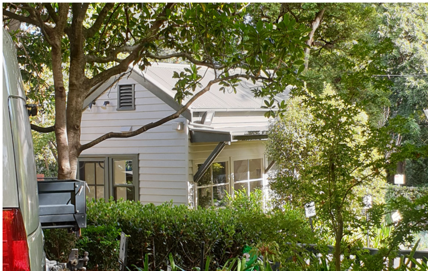
Figure 20. Former nursery. (Source: GML Heritage 2021)
