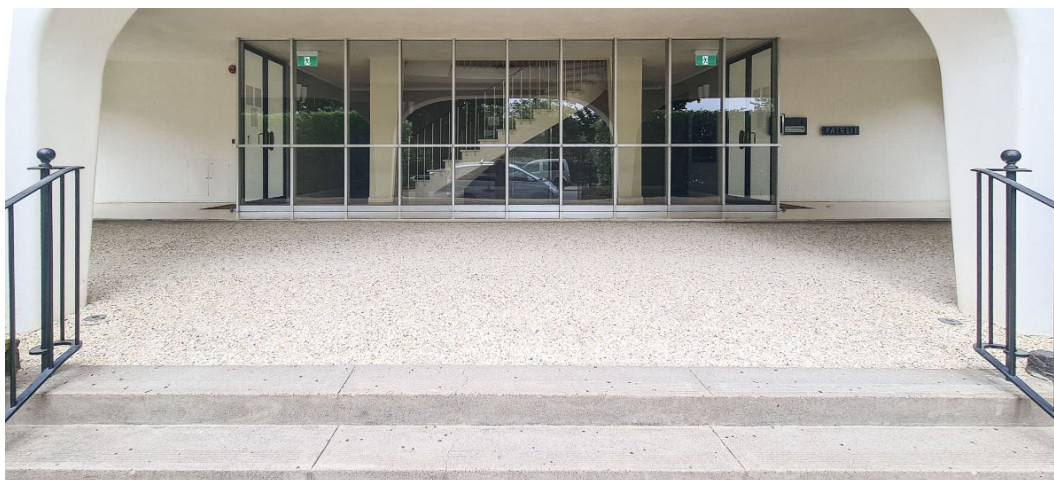
Figure 4. View of the portico and lobby enclosed by the fully glazed walls. The entrances are provided on both sides. (Source: GML Heritage 2021)
