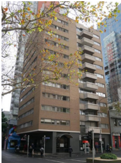
Figure 9. 287–293 Exhibition Street, Melbourne, built in 1969–71. (Source: GJM Heritage 2019)
