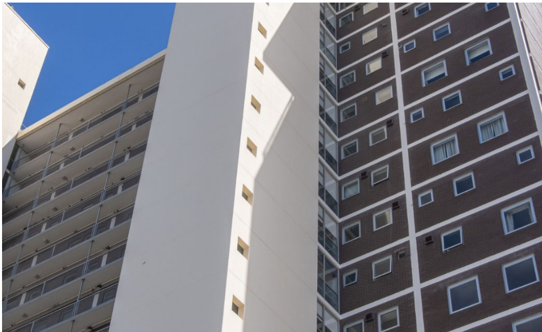
Figure 4. View of the rear elevation. Note the smaller openings on this elevation, openings on the fire staircase and the open service balconies between the service towers. (Source: GML Heritage 2021)
