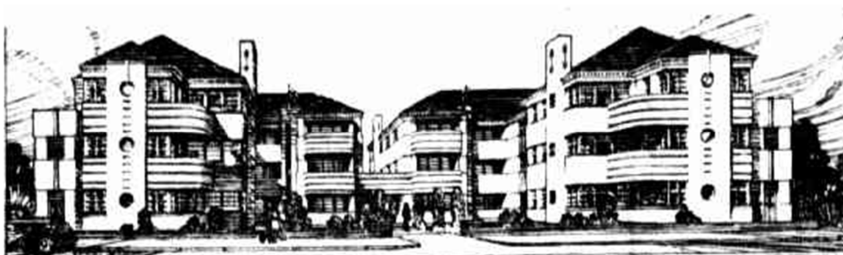
Figure 43. 'Marne Close' flats, 12–18 Marne Street, 1939. (Source: Herald , 13 December 1939:14)
