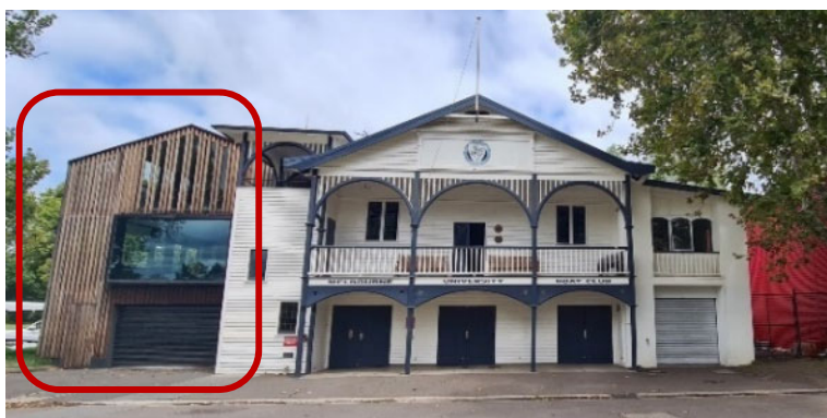
Figure 23. Principal façade of 1 Boathouse Drive, Melbourne. Note the 2012 addition in red outline. (Source: GML Heritage 2021)
