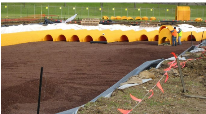
The underground storage tank is filled with arches and scoria for structural stability. This is a cost-effective method for storing water underground.
