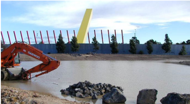
The storage wetland is excavated during construction
