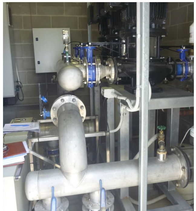
UV disinfection unit and pumps inside the pump room.
