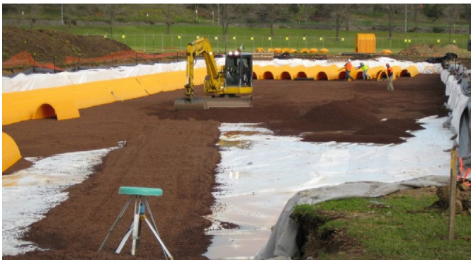
The underground storage tank during construction
